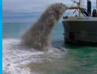
At the start of the contract 200,000m<sup>3</sup> of shingle was brought in to build up the defences. Now every year the beach is replenished by a specially commissioned dredger taking shingle from nearby banks and depositing the material at the western end of the bay
