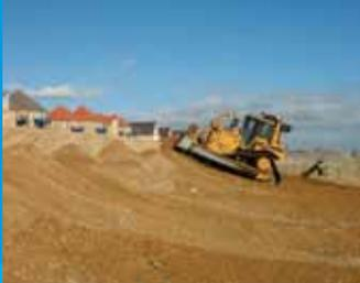
One bulldozer stays on site throughout autumn and winter to carry out day-to-day reprofiling. But if the shingle profile changes after a bad storm the contractor has to mobilise whatever plant necessary to start restoring the original shape within one tidal cycle
