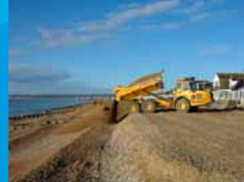
After a storm PCDL collects shingle that has been moved by the waves and returns it to the section of beach it came from. If this is done quickly enough the shingle does not dissipate over a wide area, and can be easily collected, returned and placed by bulldozer
